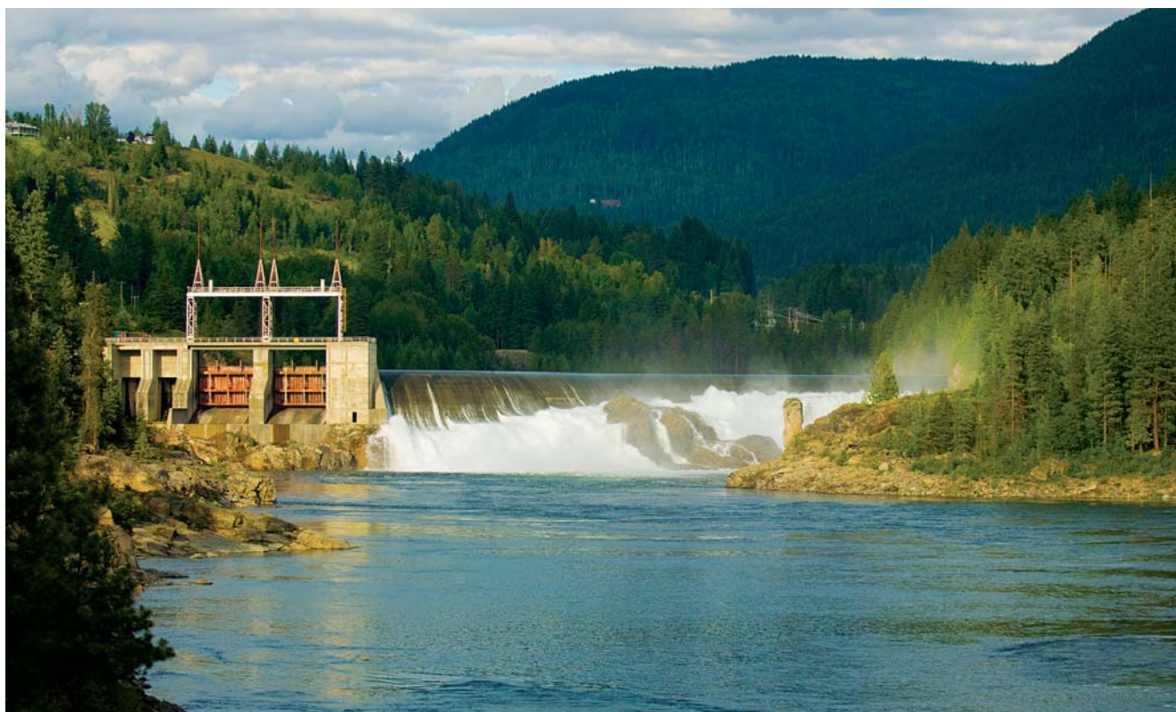
Fortis, through its regulated and non-regulated businesses, owns and/or operates 1,840 MW of generation, mainly hydroelectric.
