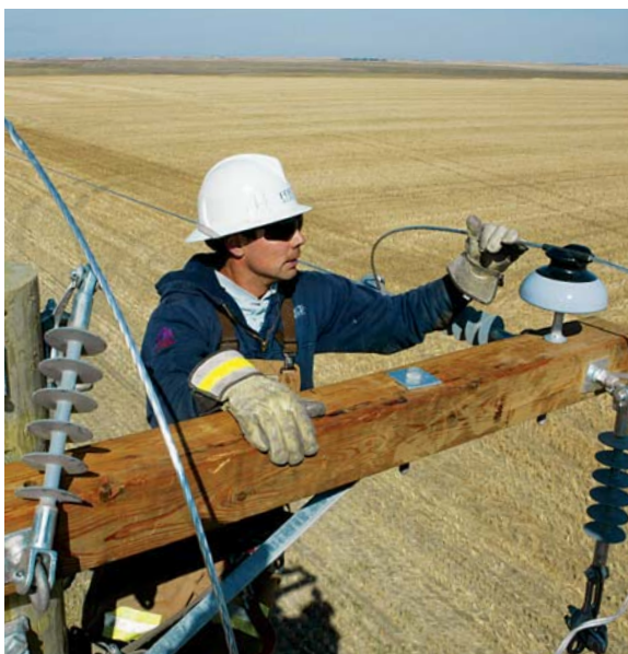
A record $407 million, before customer contributions, was invested in capital projects in 2009 to maintain the system, install automated meters and meet customer growth.
